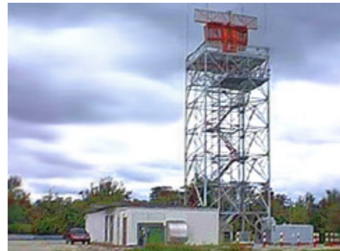
Figure 1. ASR-9 radar tower
